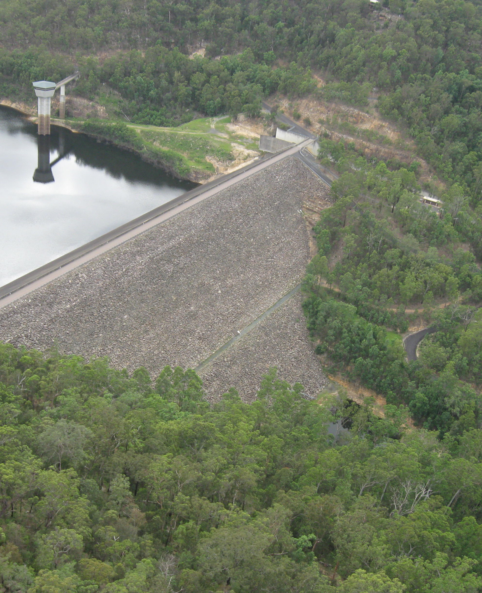
Mangrove Mountain Dam wall
