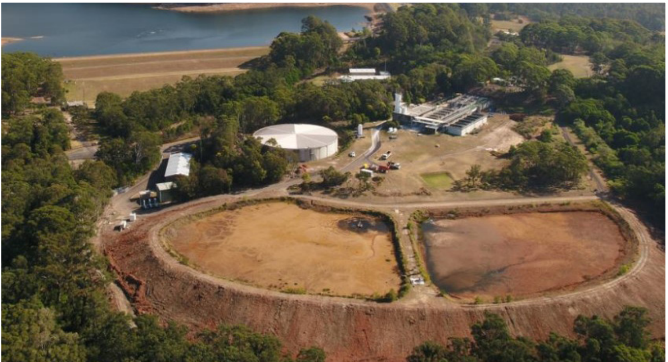
Mardi Treatment Plant - Sludge Lagoons
