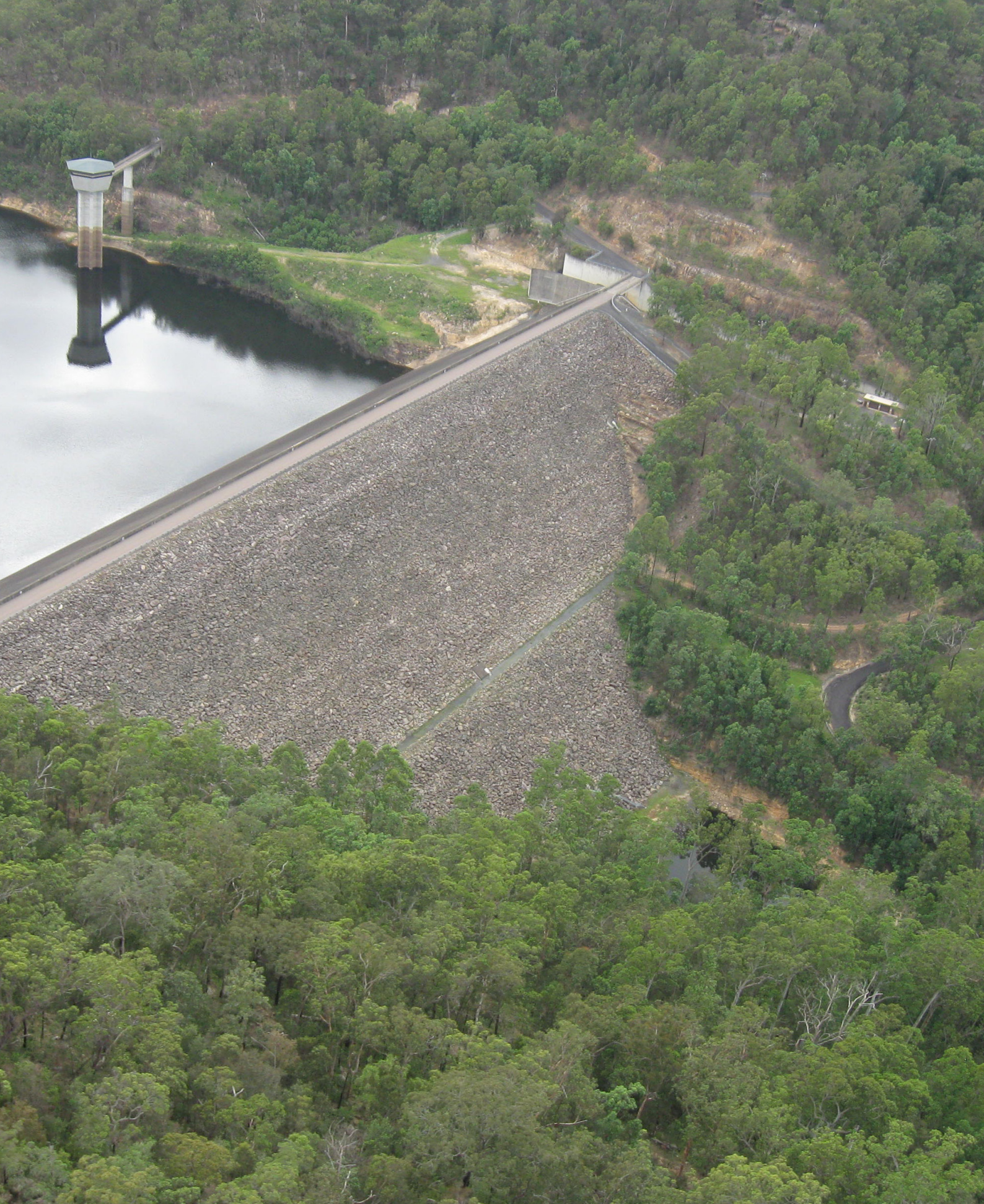
Mangrove Mountain Dam wall
