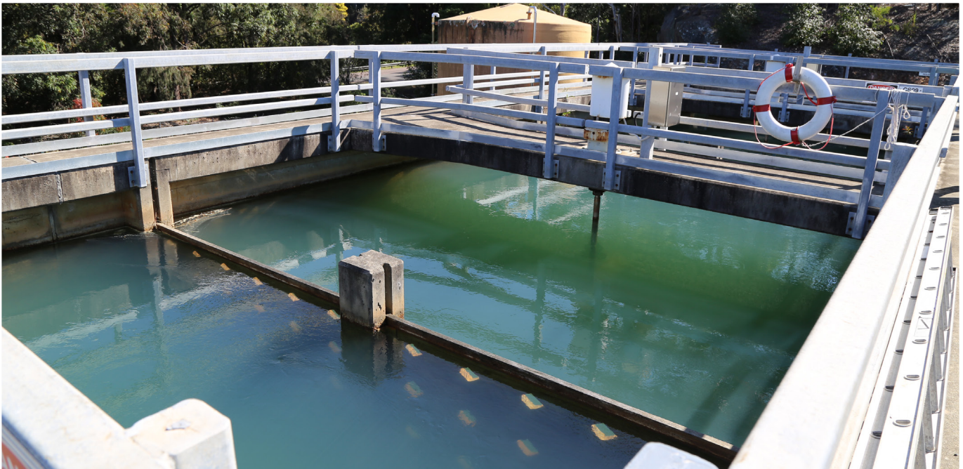
Mardi Treatment Plant - Flocculation Chamber
