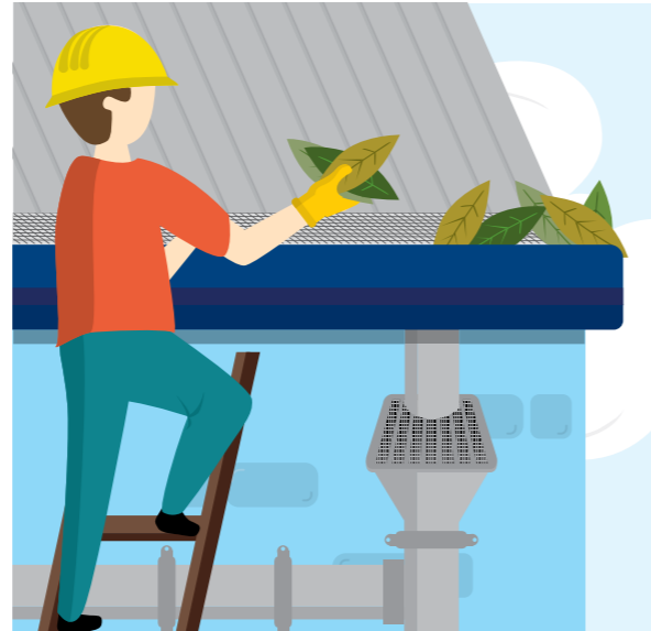
1.2 Remove accumulated leaves and debris from your roof and gutters.
